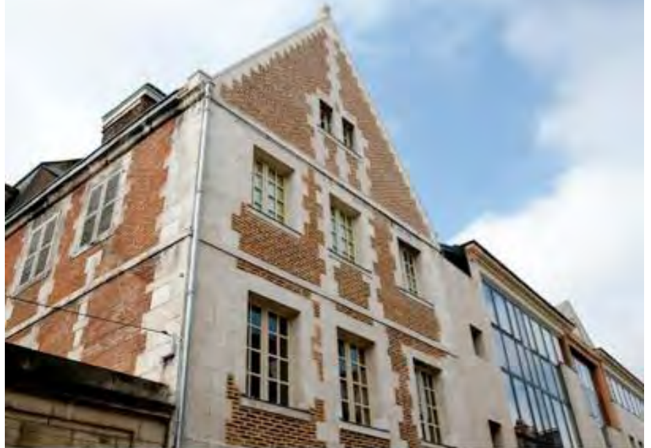
Lafarge Natural Hydraulic Lime used for pointing new build construction
