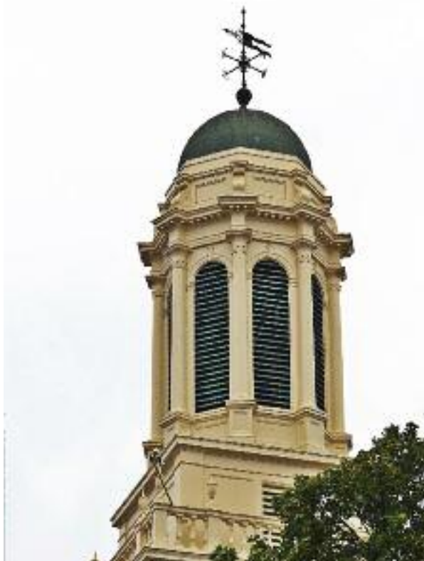
Completed Cupola Photo Courtesy Berkshire Eagle
